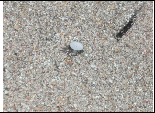
Shingle with nail sticking out
